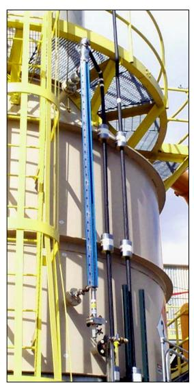
Specifically designed for low pressure, light duty applications, the new Jerguson Mini-Magnicator is a great replacement for fragile tubular glass. The Mini-Magnicator provides the same easy to read level indication as the Jerguson Magnicator, in a smaller more economical package.
